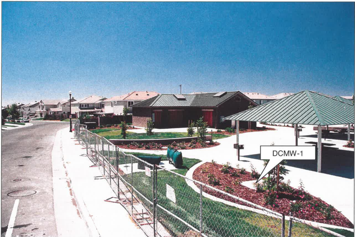
Figure 3. Photo of Diamond Creek Well Pump House and DCMW-1
